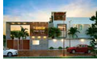
Orange Woods Near Technopark
